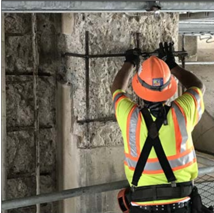
Installing rebar at Span D for concrete repair
