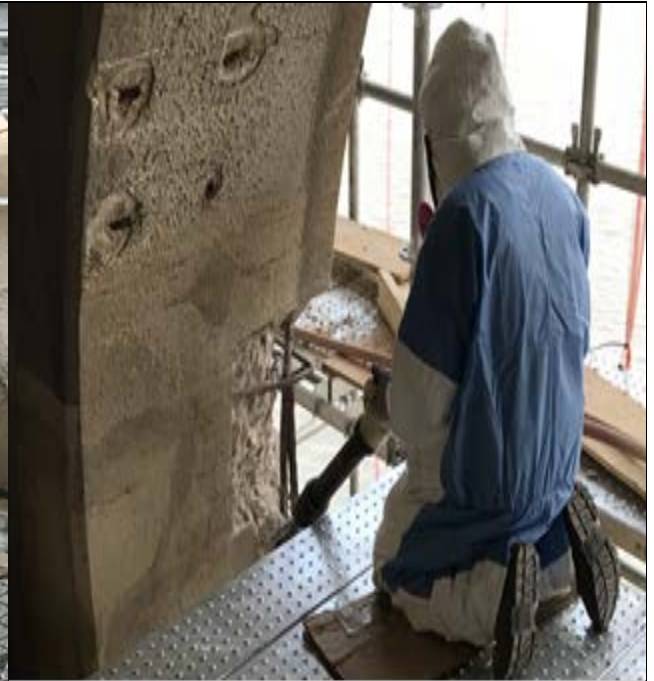
Concrete demolition at Pier 3 for concrete repair
