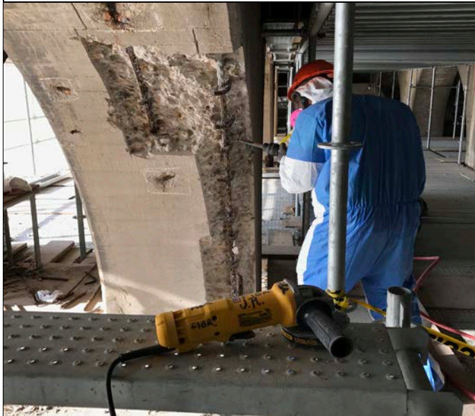
Chipping at Span D for concrete repair
