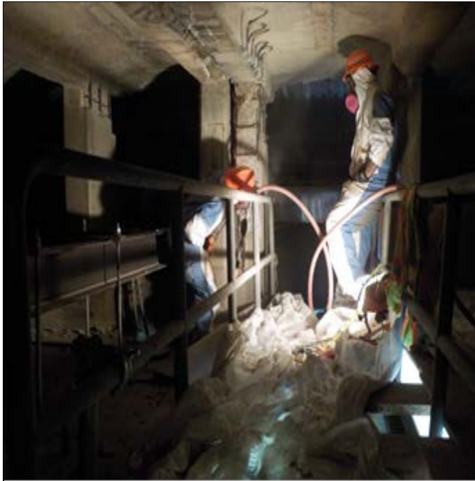
Chipping at Span C, Row D deck pedestals
