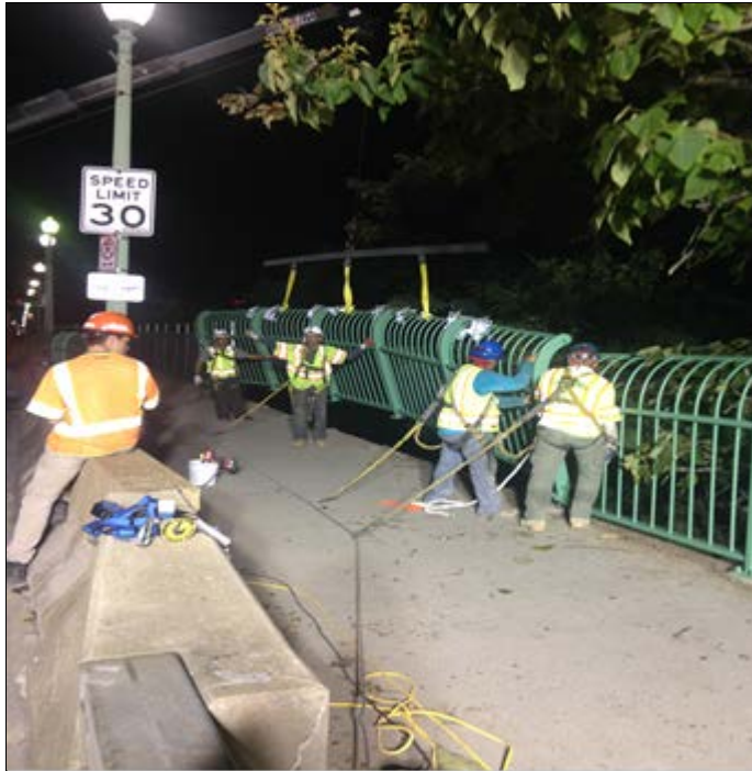
Reinstalling the pedestrian railings
