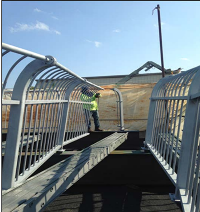
Reinstalling the pedestrian railings
