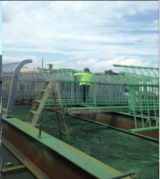
Reinstalling the pedestrian railings
