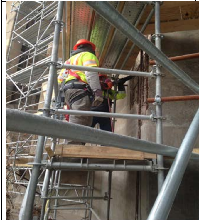
demolishing at level 7 Bent 16a East elevation North abutment
