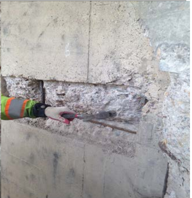
Resounding to ensure no weak concrete remains
