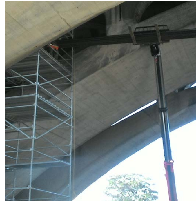
Technopref at North abutment to install air pipes
