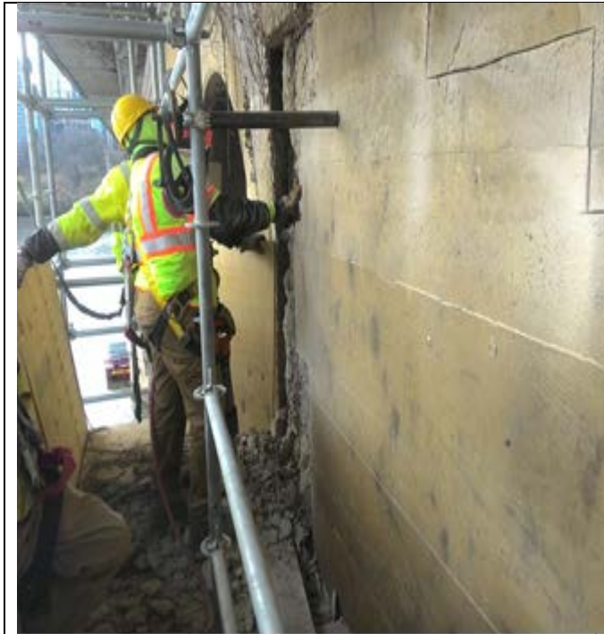
Concrete demolition at N abutment and Spandrel Arch level 2 below deck
