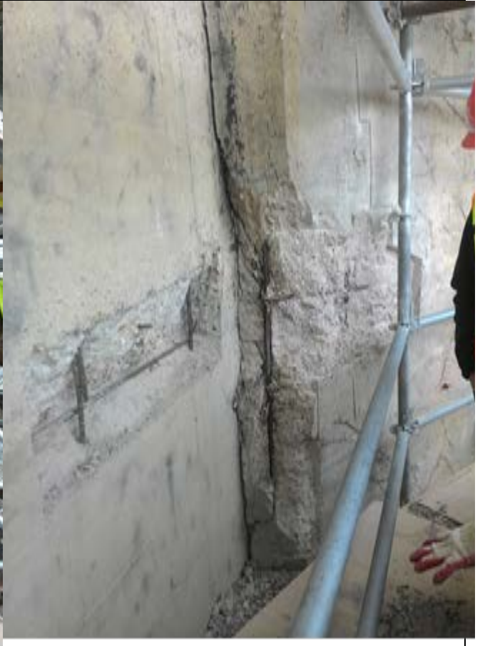
Concrete demolition on East ramp Bent 16A level 4 d
