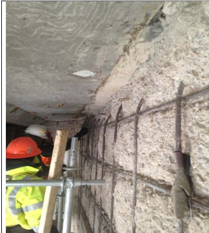
Demolishing and sounding on North abutment, East elevation
