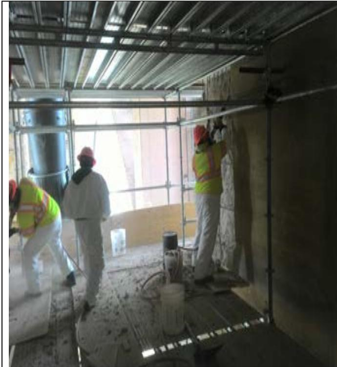
Concrete demolishing and saw-cutting at pier 4
