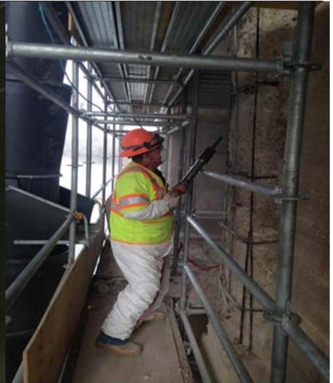
Concrete demolishing and saw-cutting at pier 4
