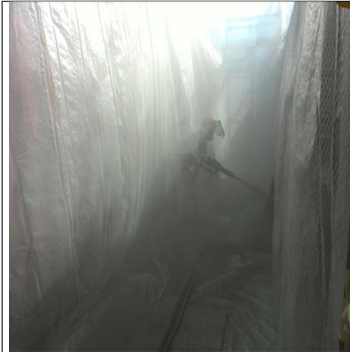
Casting 3 panels for shotcrete testing
