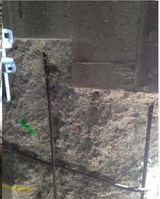
Concrete demolishing and saw-cutting at pier 4
