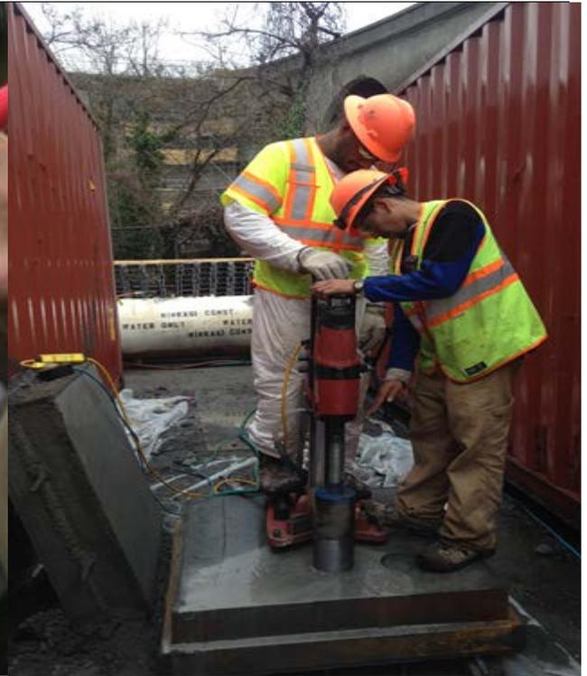
Coring concrete samples from shotcrete panels
