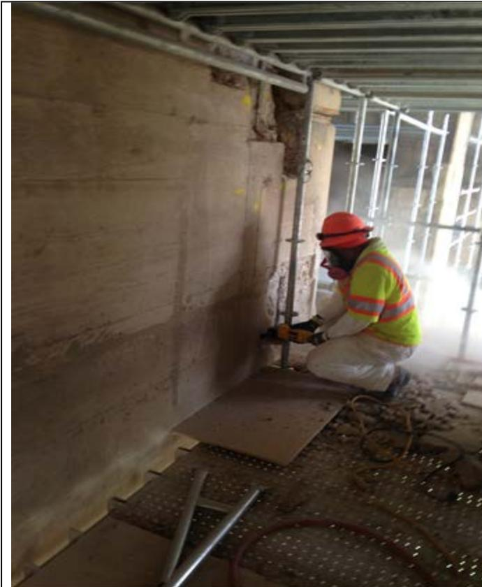
Concrete demolishing and saw-cutting at pier 4
