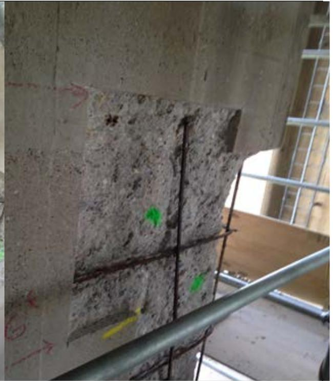
Concrete demolishing and saw-cutting at pier 4
