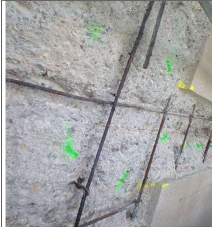
Concrete demolishing and saw-cutting at pier 4
