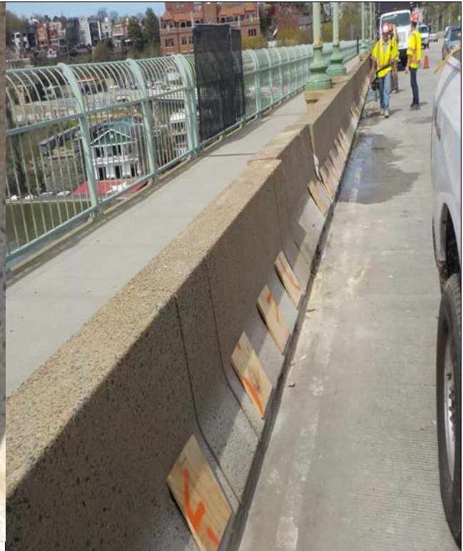
Test trial to remove and reset permanent precast concrete traffic barrier
