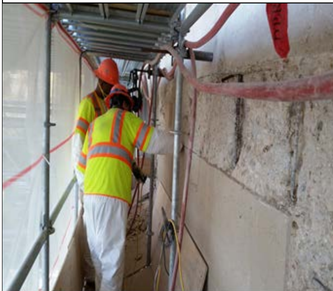
Concrete demolition at pier 4
