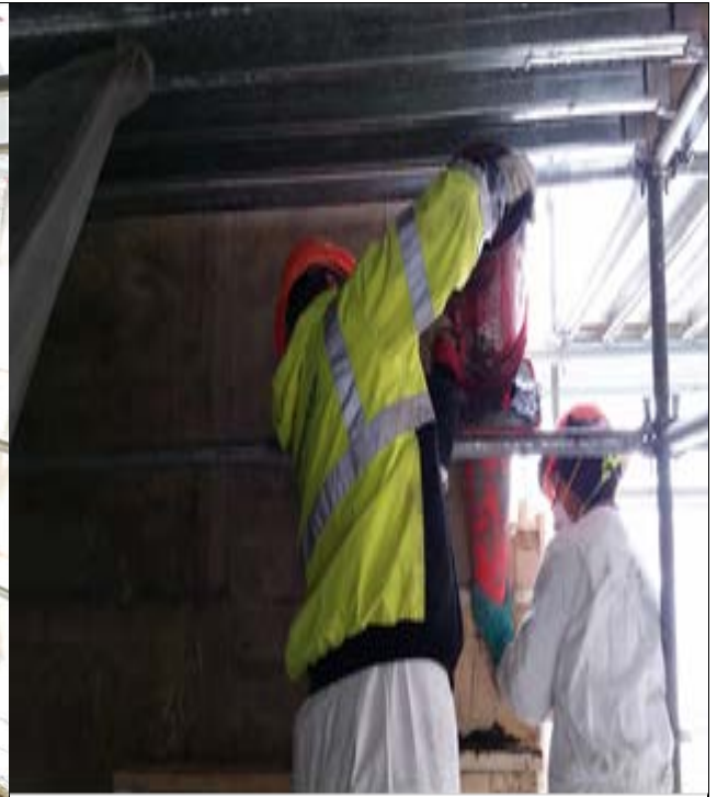
Placing concrete for concrete repairs at North abutment
