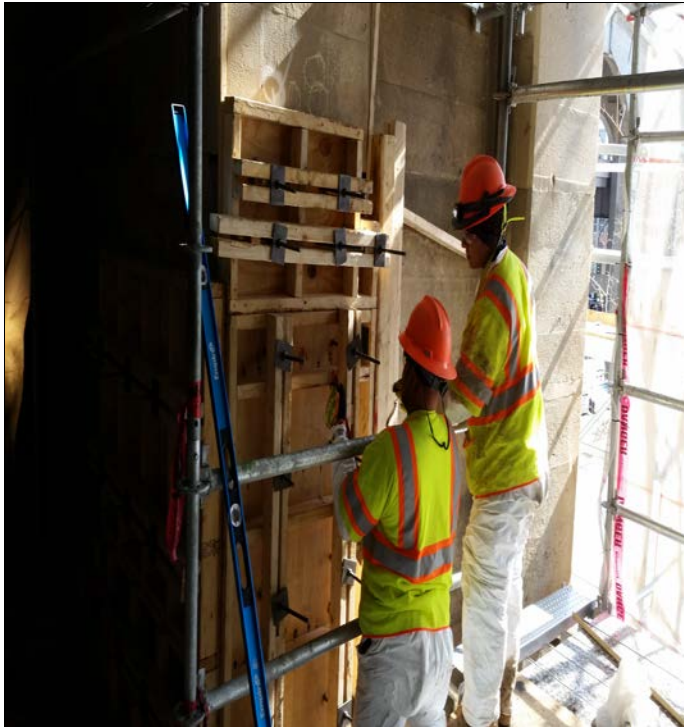
Setting up forms for concrete repair at North abutment
