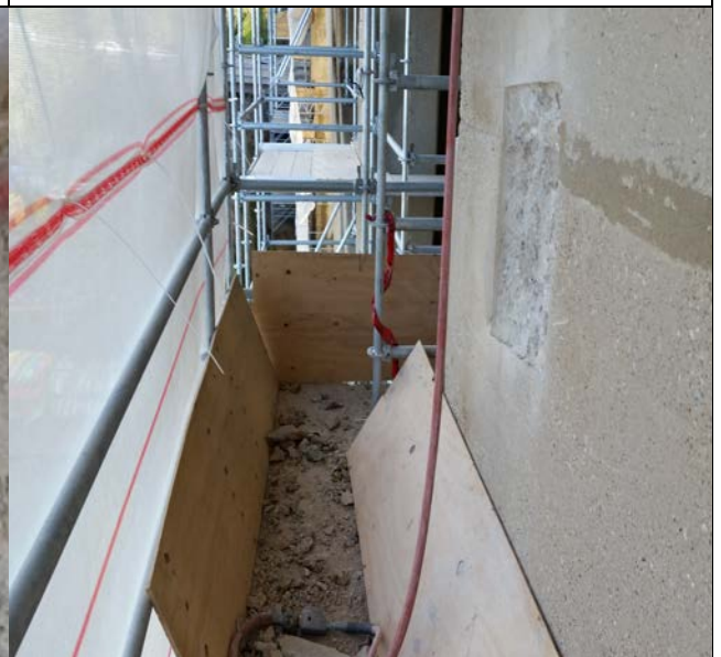
Concrete demolition at pier 4
