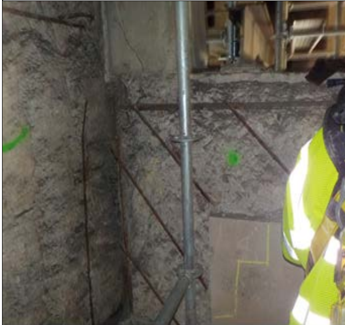
Concrete demolition at pier North abutment
