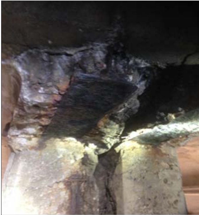
Floor beam end condition.
