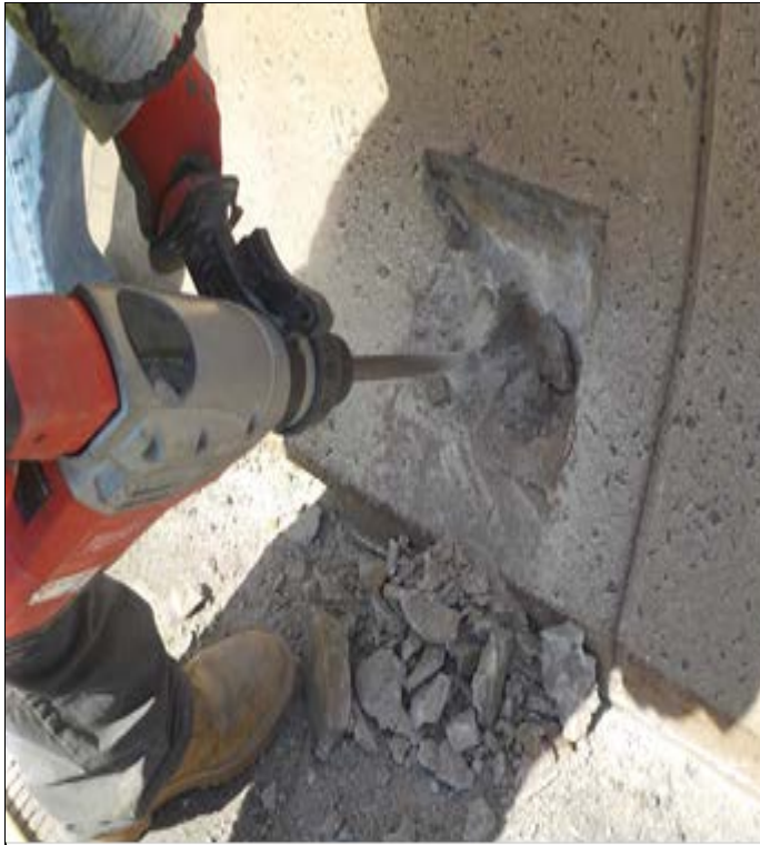
Test trial to remove and reset permanent precast concrete traffic barrier
