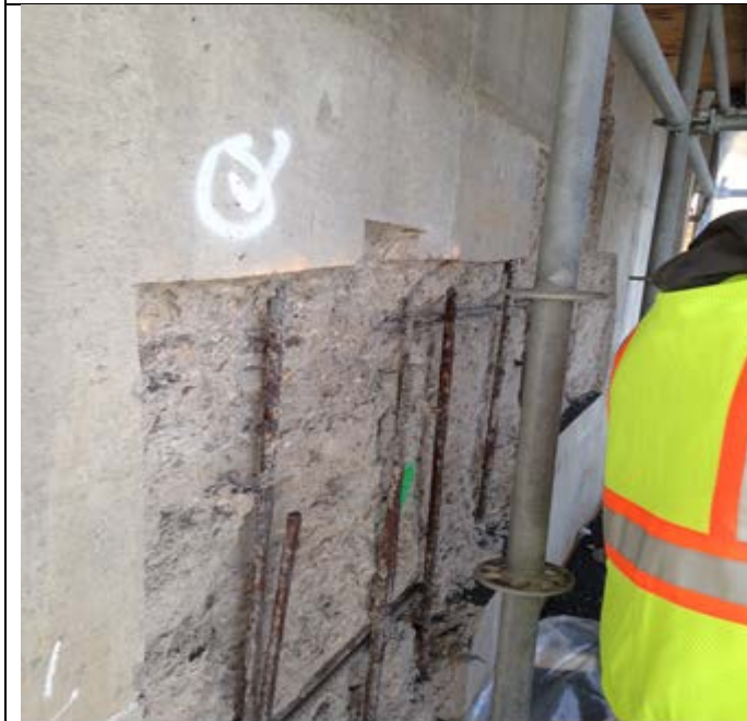
Rebar before sandblasting at Span C
