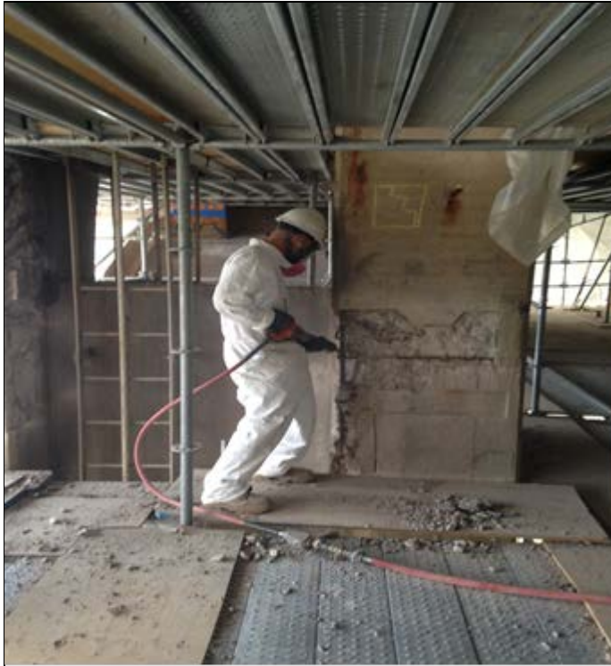
Concrete demolition at North abutment
