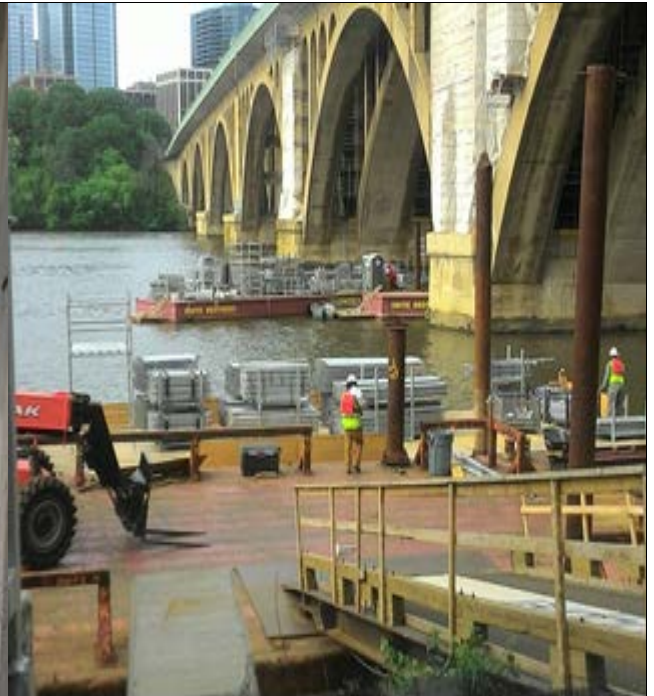
Installation of scaffold at span D
