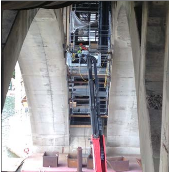
Installation of scaffold at span D
