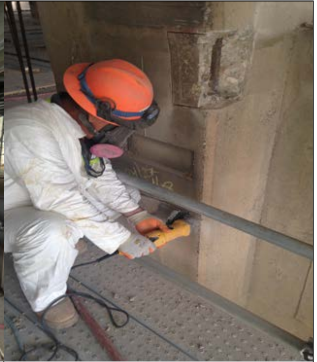
Concrete demolition and saw-cutting at North abutment
