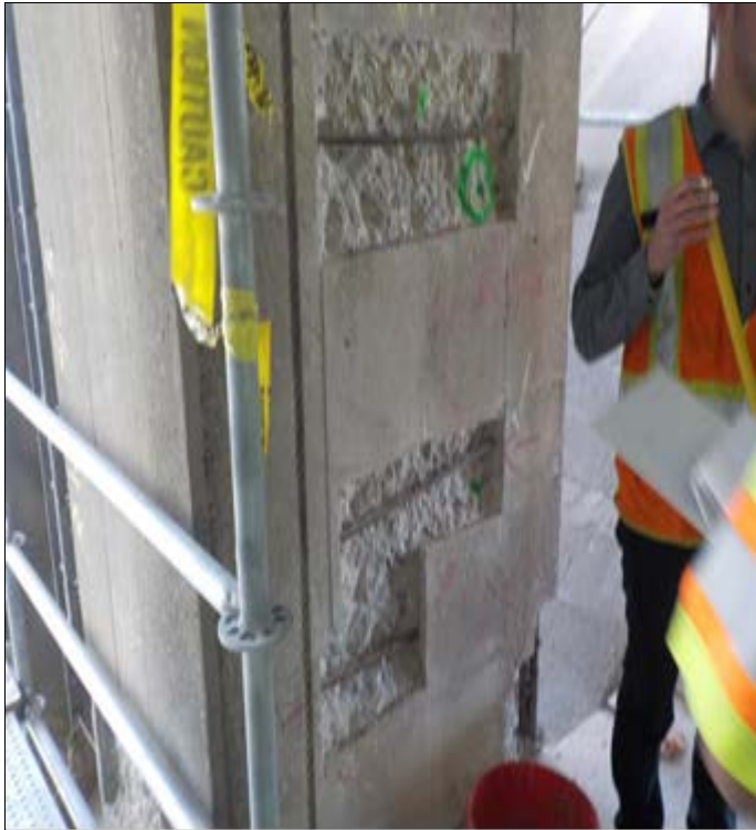
Concrete demolition at North abutment
