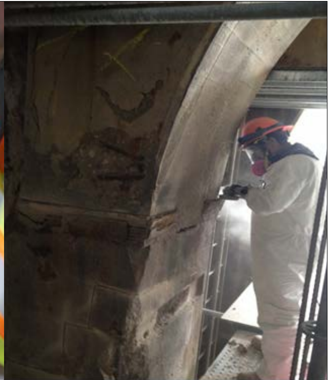
Concrete demolition at Span C
