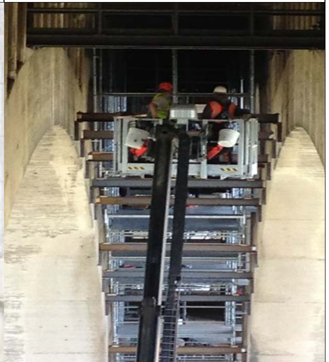
Installation of scaffold at span D
