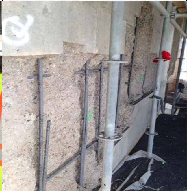
Concrete demolition and saw-cutting at North abutment
