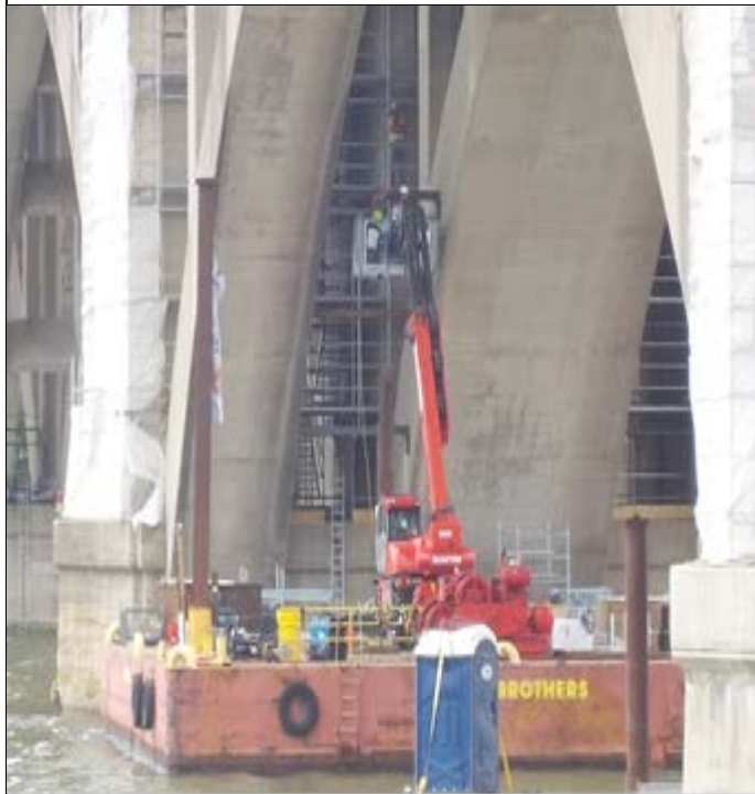
Installation of scaffold at pier 2
