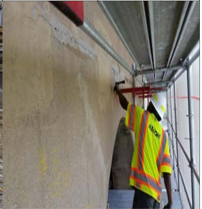
Concrete demolition at Span C
