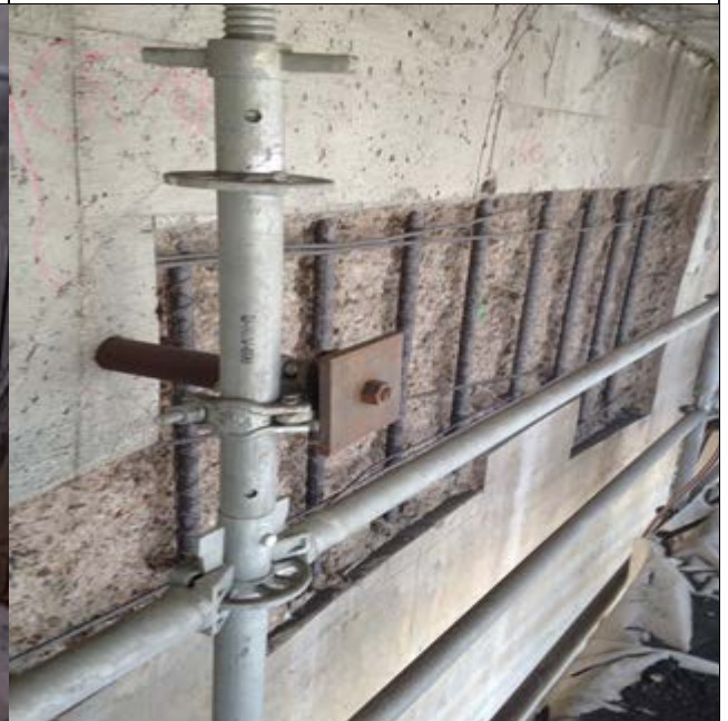
Concrete demolition and saw-cutting at North abutment
