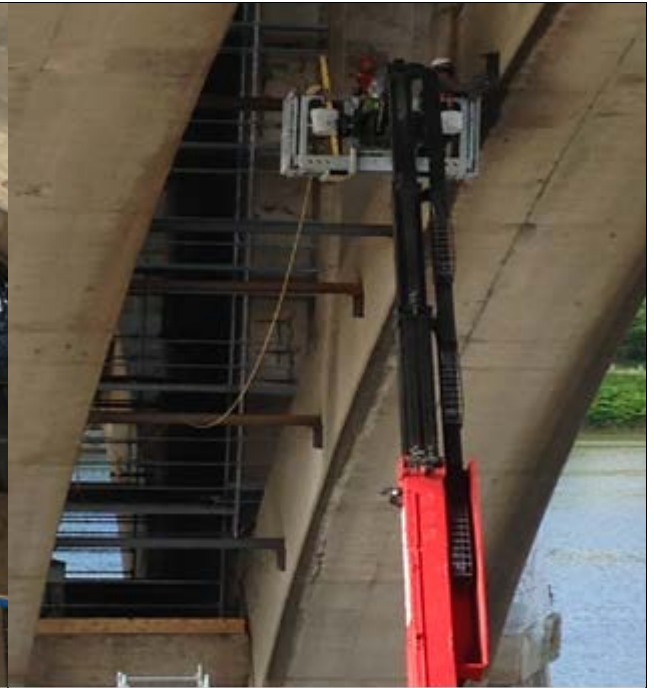
Installation of scaffold at span D
