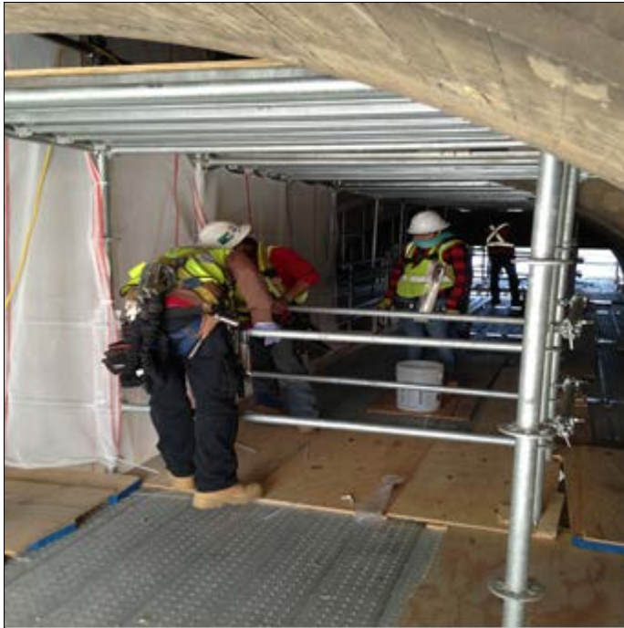
Installation of scaffold at span D
