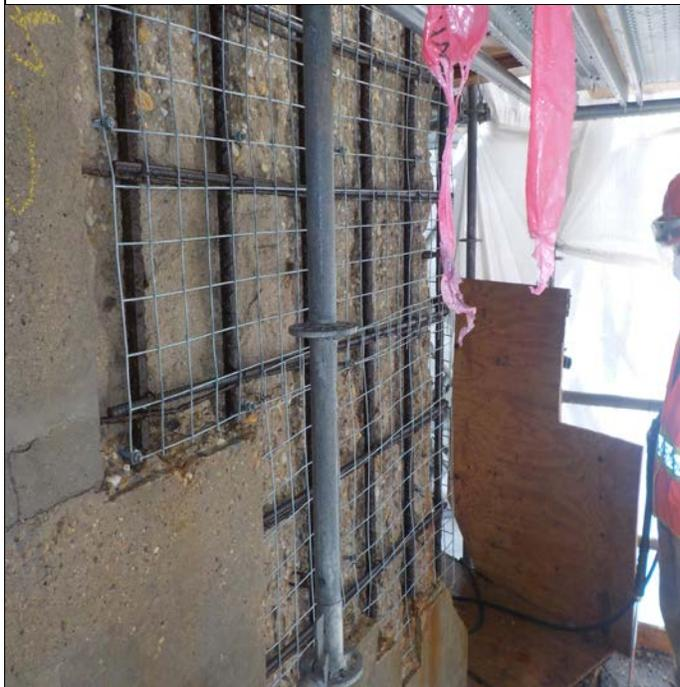
Installation of anchors and wire mesh for type 1 repair at North abutment
