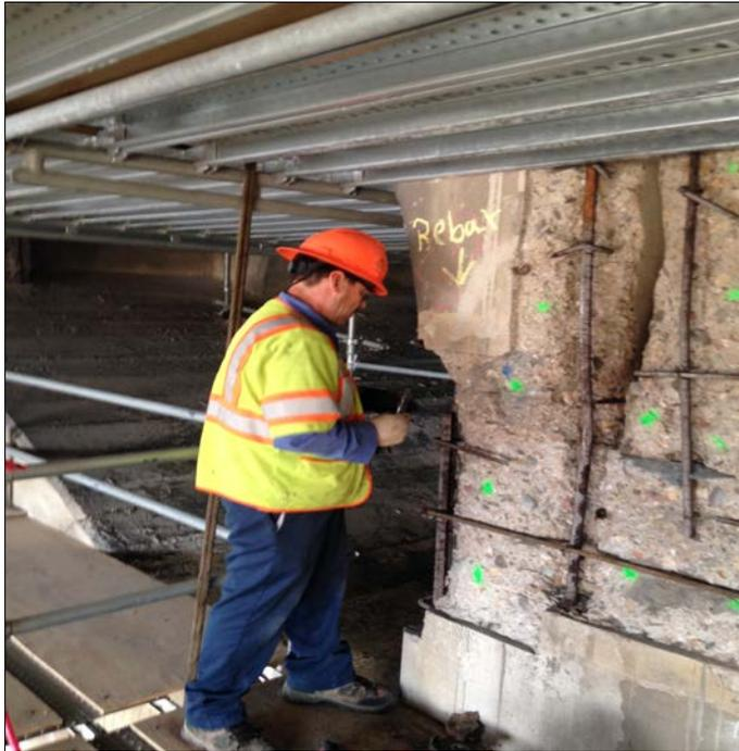
Concrete demolition at span C.
