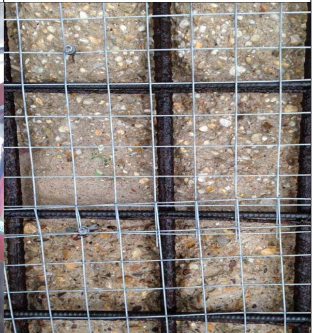
Installation of anchors and wire mesh for type 1 repair at North abutment
