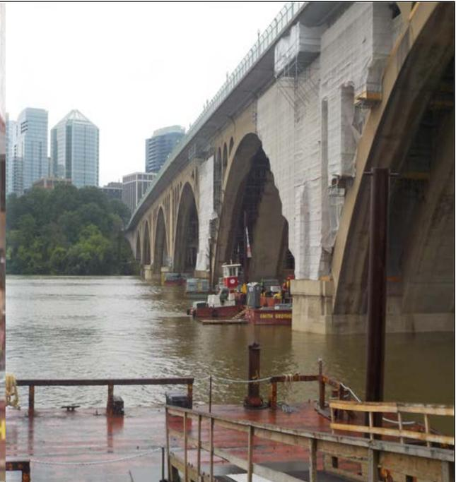
Installation of scaffold at span D
