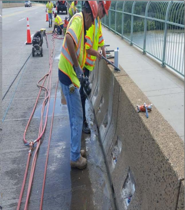
Remove and reset permanent precast concrete traffic barrier
