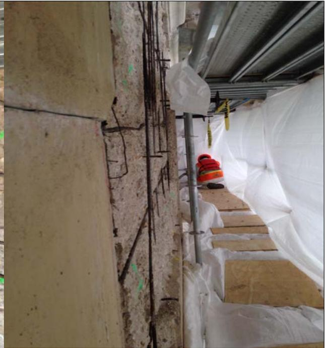
Concrete demolition and installation of containment.
