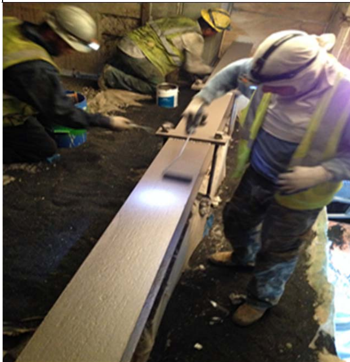
Painting operation for the water main beams
