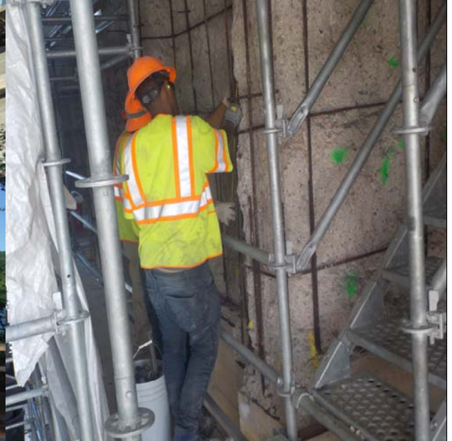
Chipping and saw-cutting for concrete repairs
