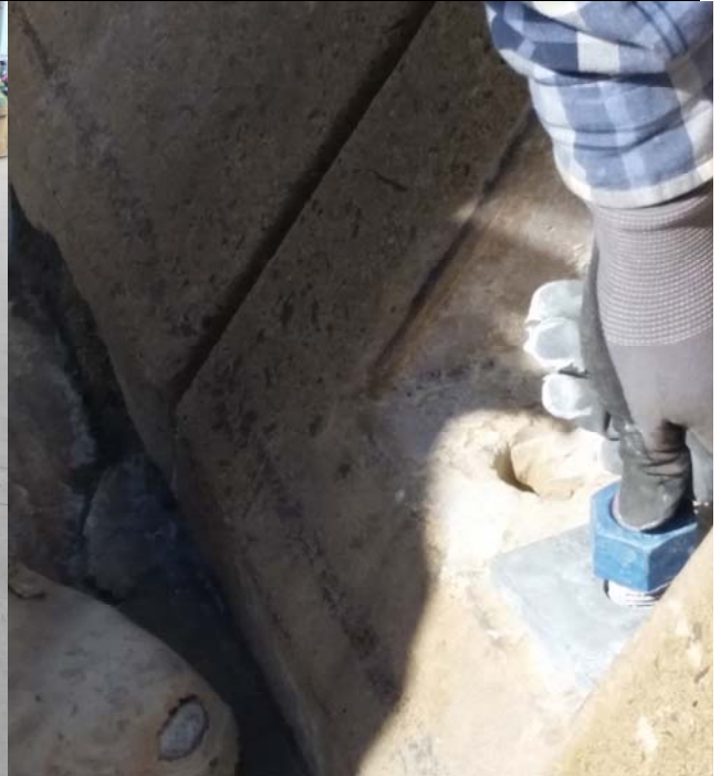
Remove and reset permanent precast concrete traffic barrier
