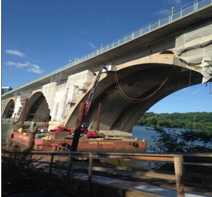
Chipping and saw-cutting for concrete repairs
