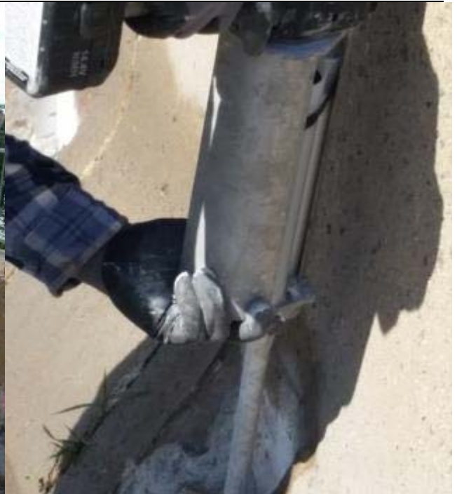
Remove and reset permanent precast concrete traffic barrier
