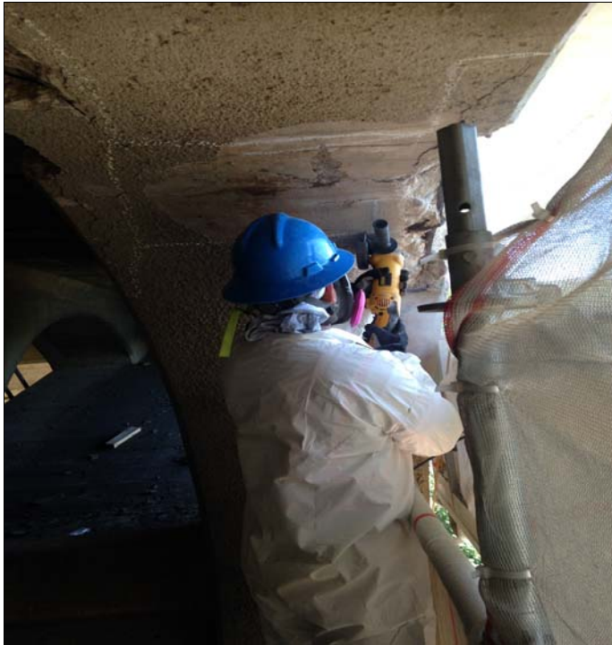
Chipping and saw-cutting for concrete repairs
