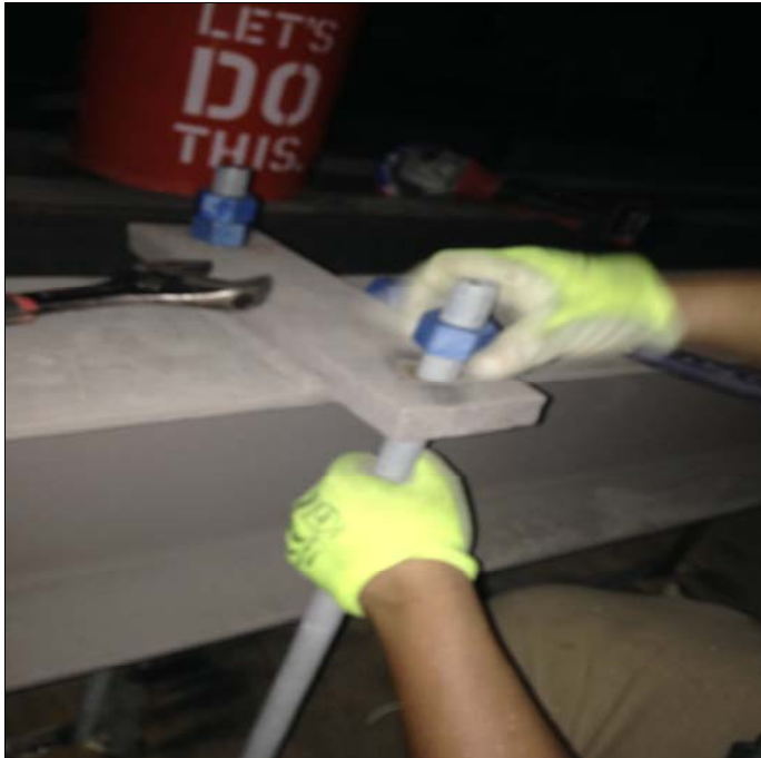
Installing anchor rods for the water main support beam
