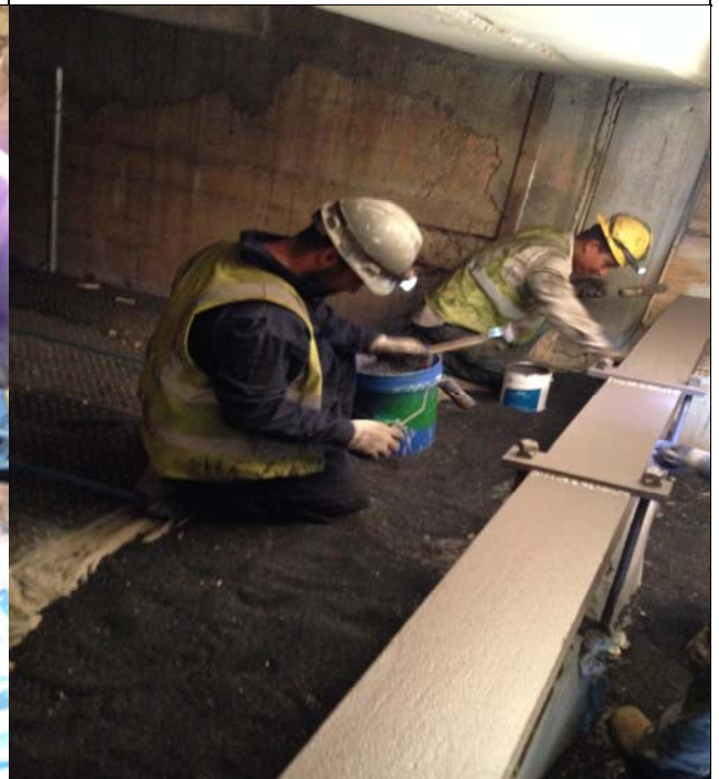
Installing anchor rods for the water main support beam
