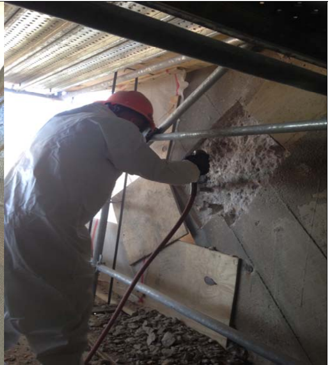
Chipping and saw-cutting for concrete repairs
