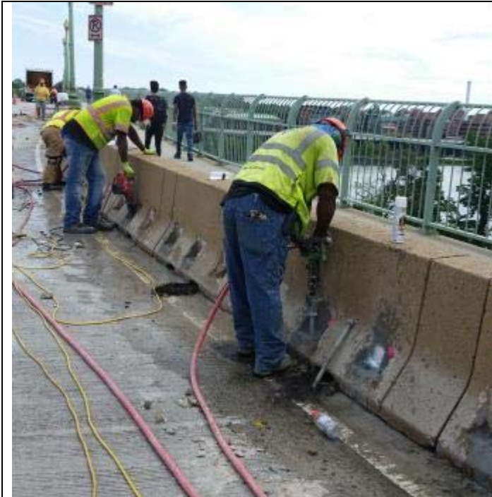
Remove and reset permanent precast concrete traffic barrier
