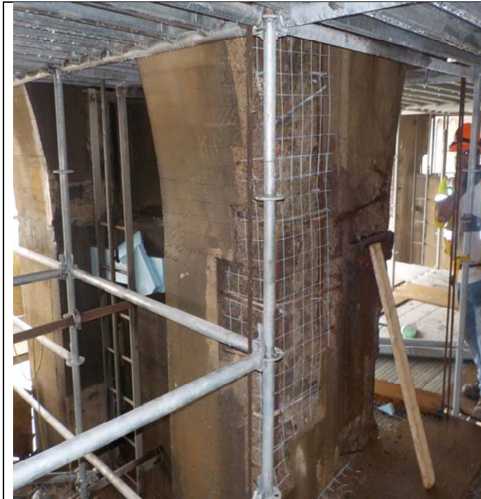
Installing rebars and wire mesh for concrete repair
