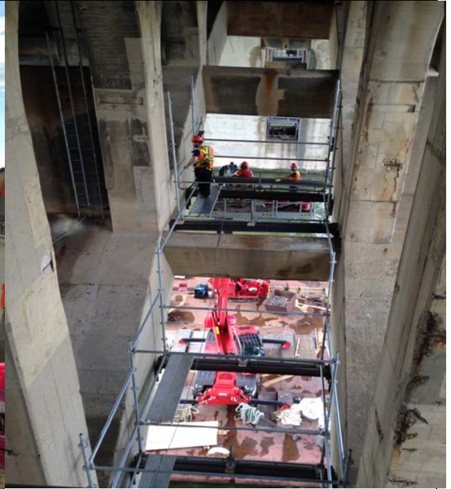
Installing scaffold system
