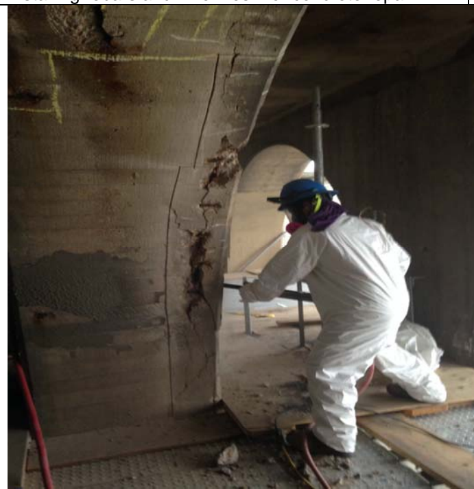
Chipping and sawcutting for concrete repairs
