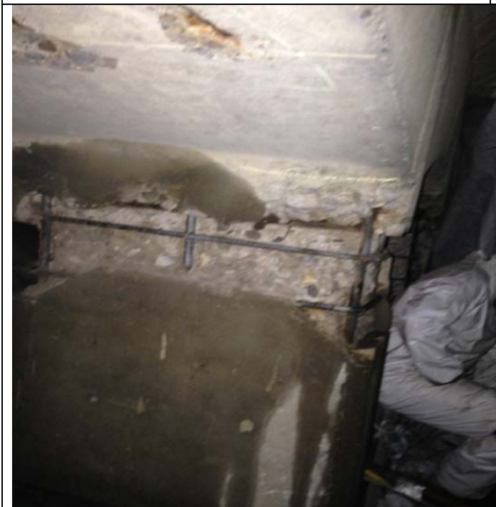
Repair deck pedestal operation
