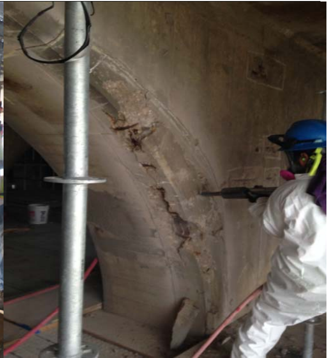
Chipping and saw cutting for concrete repairs
