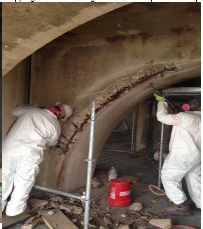
Sounding and marking locations for concrete repair
