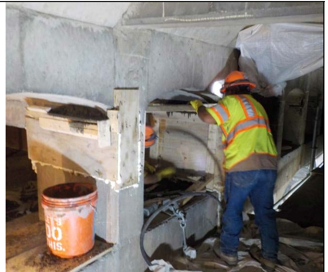
Fibrowrap placing Sika 211 concrete Form & Pour to deck pedestals Floor Beams 12-15
