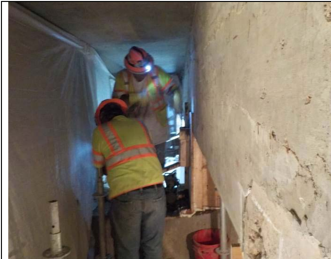
Fibrwrap placing Sika 211 concrete Form & Pour to deck pedestals Floor Beam 7, Row C
