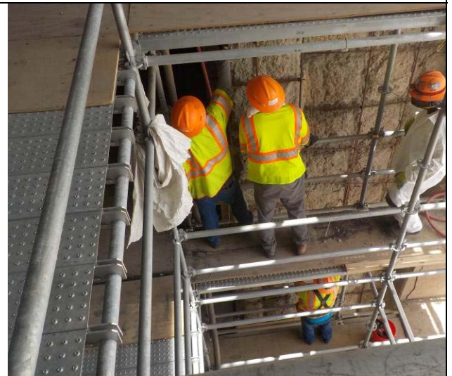
Fibrowrap placing Sika 211 concrete Form & Pour to deck pedestals Floor Beams 12-15
