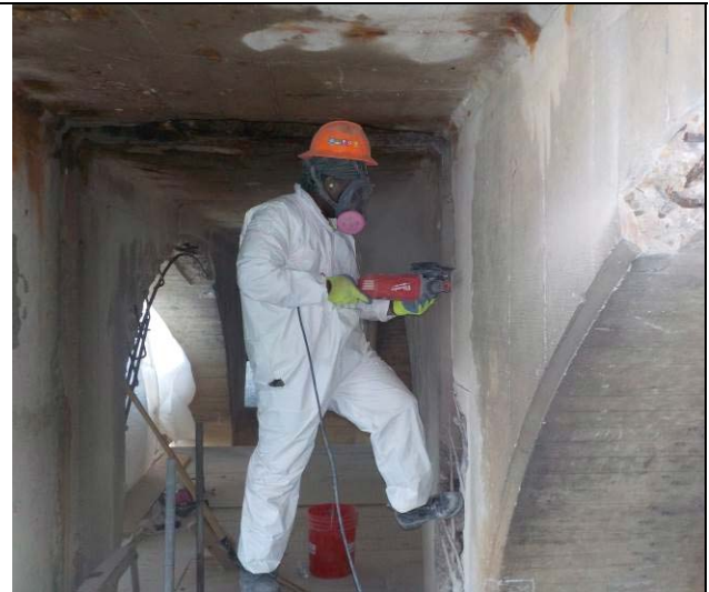
Fibrwrap saw-cutting and demolition on Span C, Row A, Columns 10-11, E face near Pier 4, Level 2
