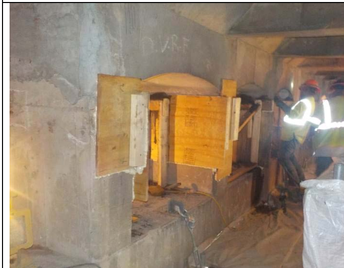
Fibrwrap placing Sika 211 concrete Form & Pour to deck pedestals Floor Beams 7-12
