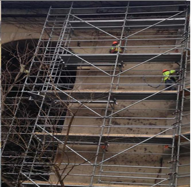
Sounding, marking and demolition activities on North abutment, East elevation and
