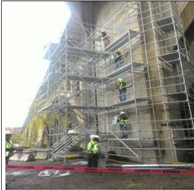
Scaffolding erection at N. abutment.
