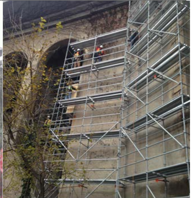
Erecting scaffold system at North abutment
