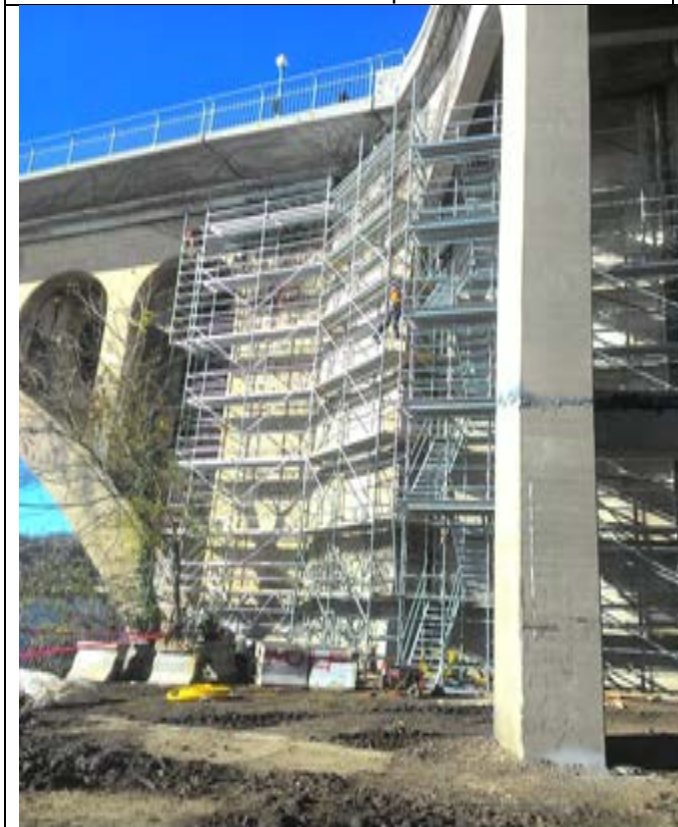
Erecting scaffold system at North abutment
