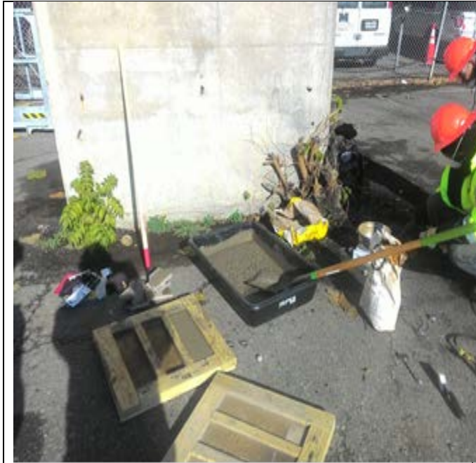
Fibrwrap color matching samples with Sika 211 Sample at Bent 16A
