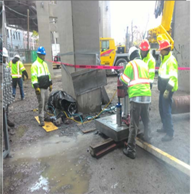
Fibrwrap core test samples from Test Panel at N. Abutment on East Ramp, Bent 16A
