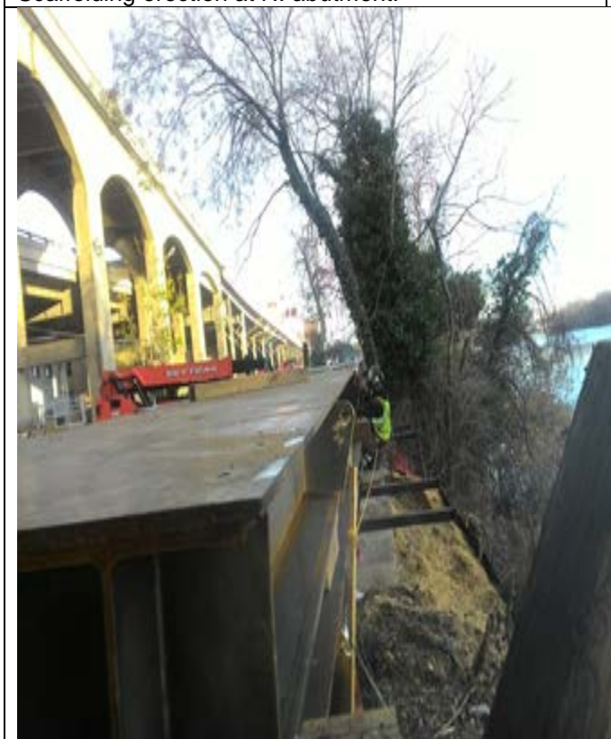
Assembling sections of the water access ramp
