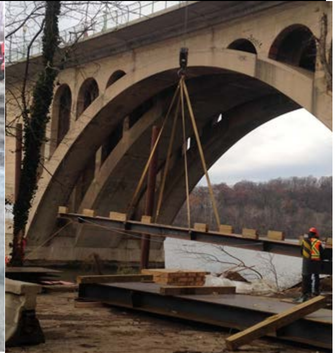
installation of water access ramp
