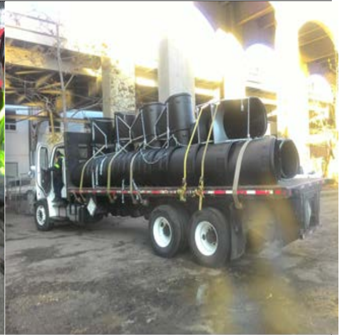
Technopref received Chutes for debris
