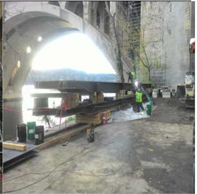
Assembling sections of the water access ramp
