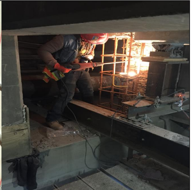
Demolition work for Span D Deck Pedestal A49, which is a full replacement
