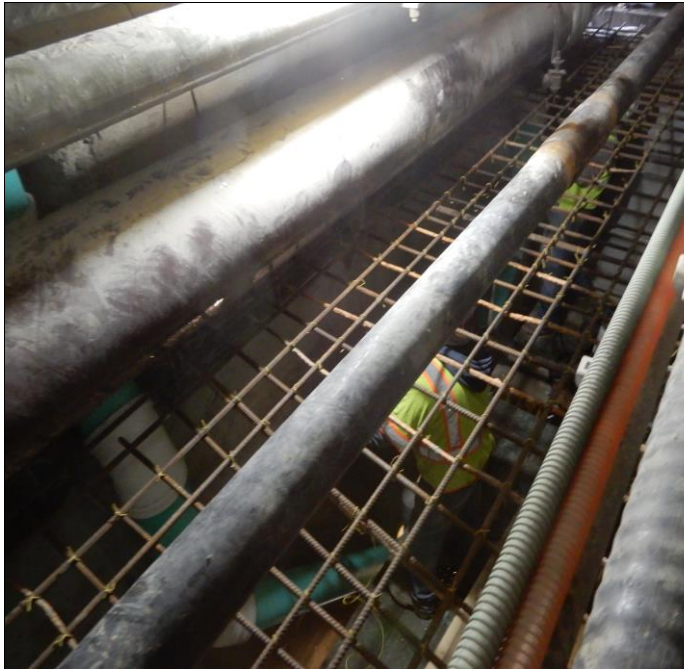
Installing rebar and forming the East Gallery floor slab at Pier 4
