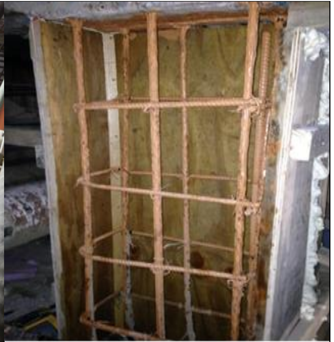
Formwork for Span D Deck Pedestal A49, which is a full replacement
