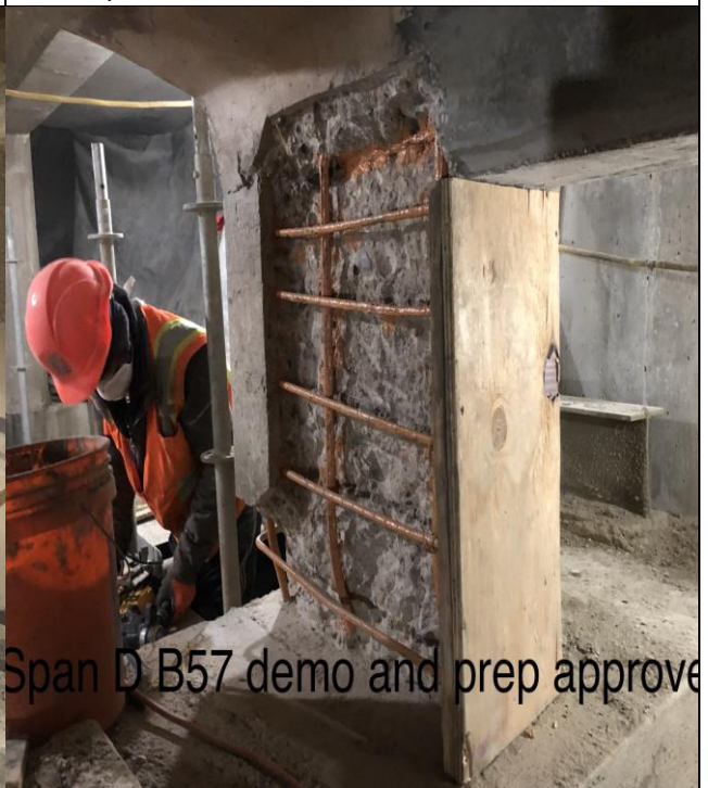
Demolition work for Span D Deck Pedestal A49, which is a full replacement
